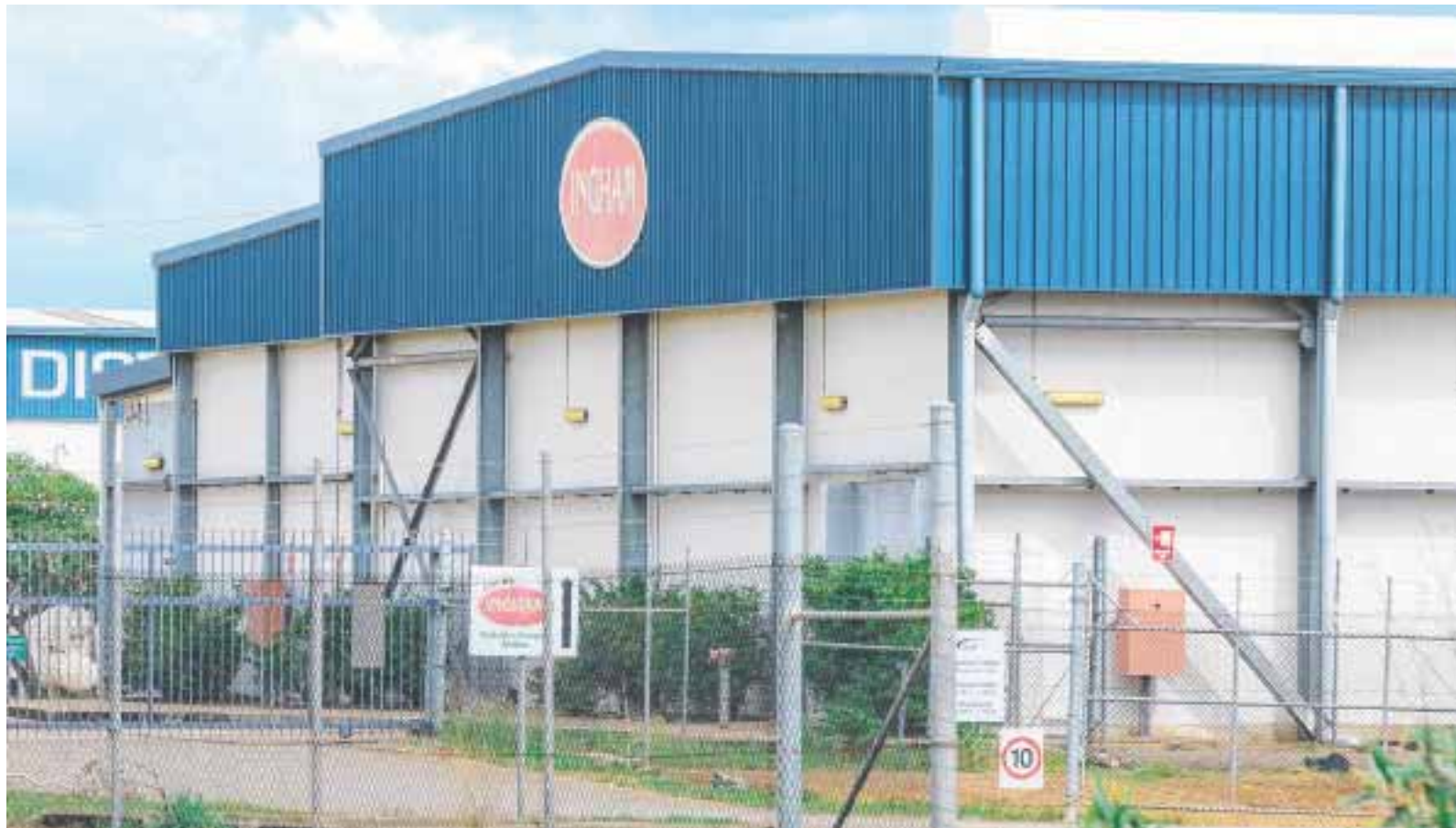
Sentinel Property Group bought Ingham's Group cold storage facility at Wishart for $7.4m. Picture: Glenn Campbell
