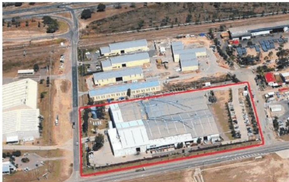
Sentinel’s newly-acquired industrial facility (outlined) at 806 Ingham Rd, Bohle.
