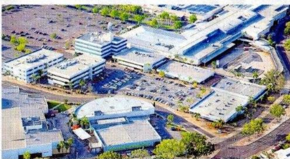
NEW BRANCH: STEPS has leased a 416sq m office at the CasCom Centre at 13-17 Scaturchio St, Casuarina, in the Northern Territory. PHOTO: CONTRIBUTED
