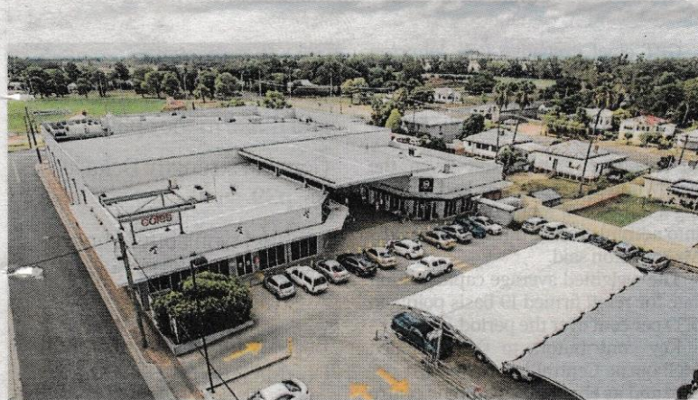
Sentinel's Gunnedah Shopping Centre in north-west NSW.
